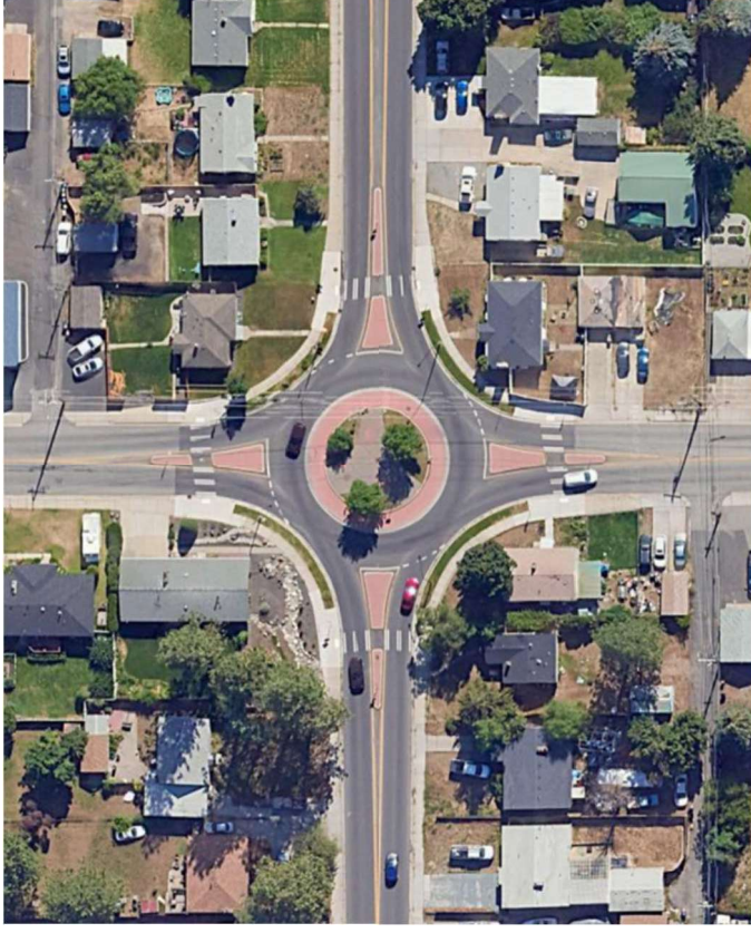
Exhibit 6.1. Wellesley Avenue & A Street Roundabout
