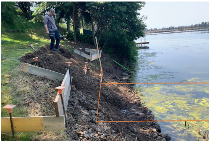
Photo 6 Early stage of construction
