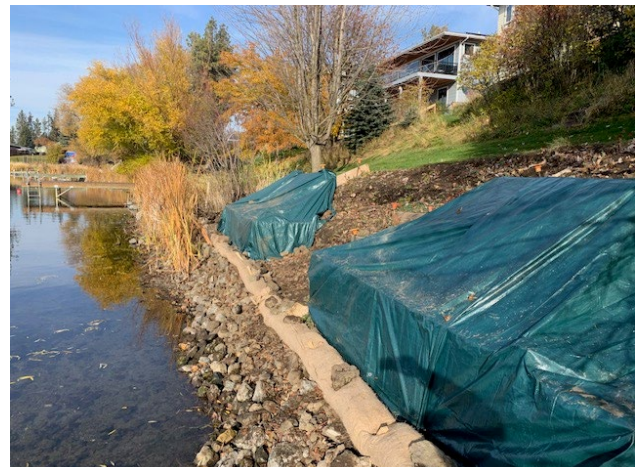
Photo 7 Secured site in 2025 prior to winter, with fiber wattles and tarps
