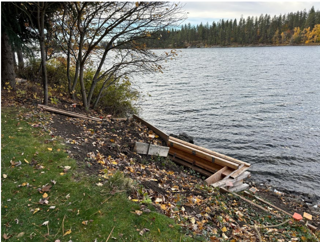
Photo 4 OHWM and forms installed facing south west
