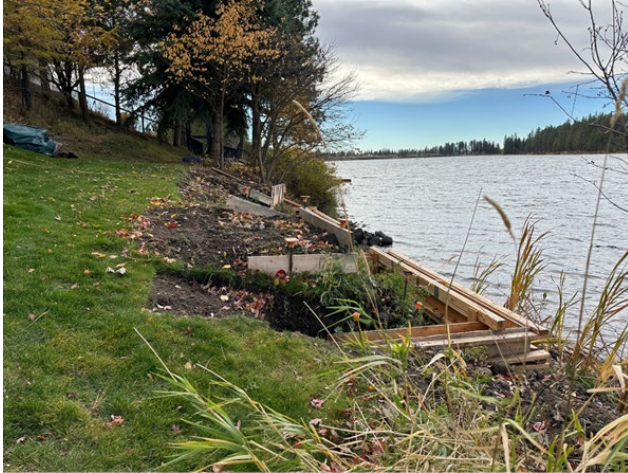
Photo 2 Forms for Bulkhead/landings to the proposed dock
