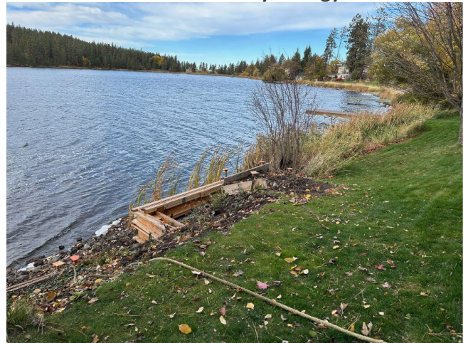
Photo 5 OHWM and forms installed facing northwest
