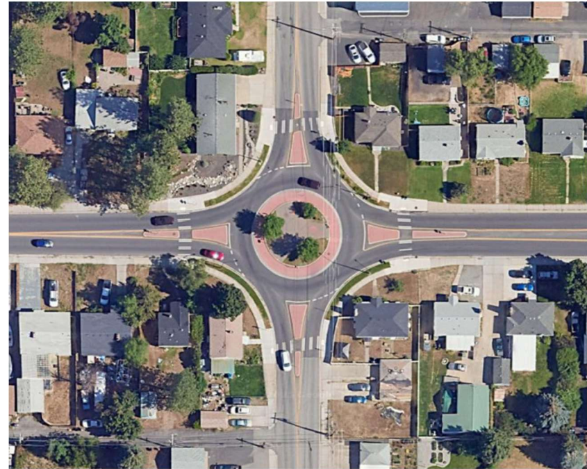
Exhibit 6.1. Wellesley Avenue & A Street Roundabout
