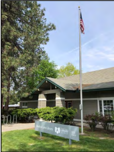
Image 5.2 Public Library Facility
