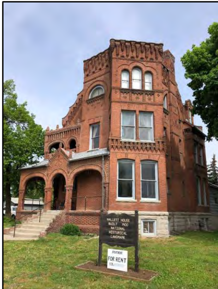
Image 7.1 Historic Hallett House
